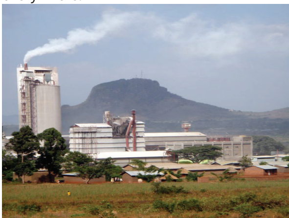
Fig. 4.2: Tororo cement works. It uses limestone from the quarry behind
